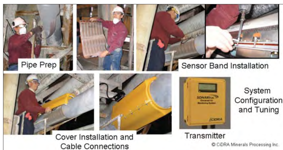
Figure 1. Installation procedure from (top-left) pipe preparation through cleaning and light sanding of pipe to (top-middle and top-right) mounting of the flexible, lightweight sensor band to (bottom-left) installation of the sensor cover and to (bottom-middle and bottom-right) connection of sensor cover to transmitter via water tight cable
